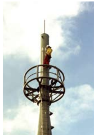
ABOVE LEFT. Vertical fall arrest system installation, Northland. ABOVE RIGHT. Line testing at Te Papa Museum, Wellington.
