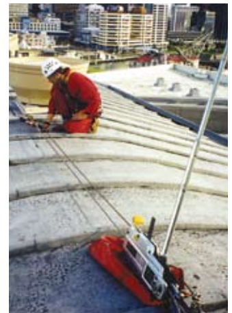
ABOVE LEFT. Vertical fall arrest system installation, Northland. ABOVE RIGHT. Line testing at Te Papa Museum, Wellington.
