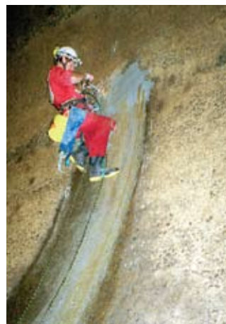
ABOVE LEFT. Concrete repairs, Aratiatia Intake. ABOVE RIGHT. Rock anchoring, Arapuni.
