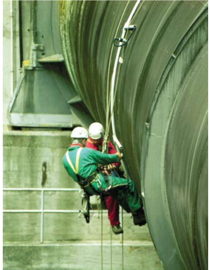
ABOVE. Penstock transducer replacement, Maraetai.
